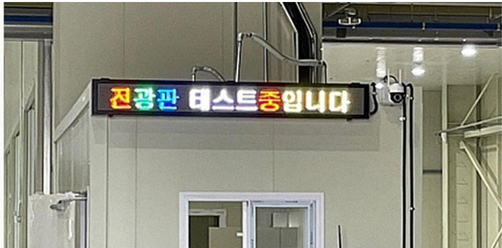
LED Display Board, CCTV
